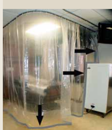
FIGURE 17 Plastic curtain taped to wall.
