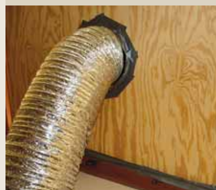
FIGURE 6 Flex duct connected to window template. The other end of the flex duct should be connected to the HEPA machine.
